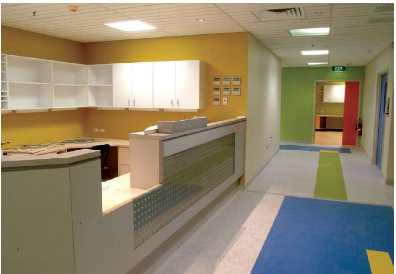
Partially completed nurses base for JSAOU. Note interior design scheme
