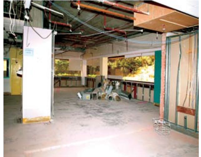
Demolished Ward 3B
