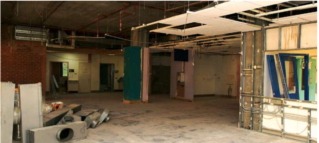
Completed Demolition of the Original Ward 3B
