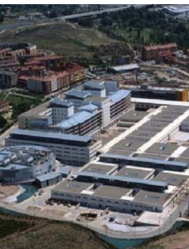
Hospital San Pedro - Antonio Menendez Metreveli Deputy Director for Infrastructure and technical services
