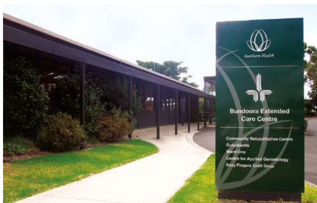
Bundoora Extended Care Centre
